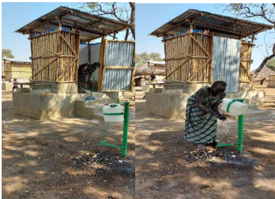
Nyawuor Ter, South Sudanese refugee, cleans latrine and washes her hand installed pedal tippy tap near the latrine in her compound in Nguennyiel camp Gambella Ethiopia,
