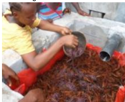
Adding worms to tiger worm vermi filter toilet system in Monrovia, Liberia. The worms consume the faecal waste negating the need for emptying
