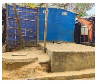
Figure 7: Septic tank with soak pit example
