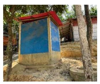
Figure 4: Direct pit with offset soak well single cubicle latrine example
