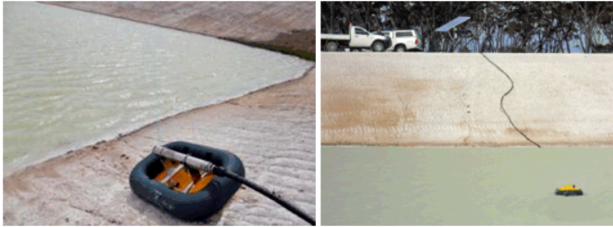
Fig 9: Submersible pump installed on a floating pontoon
