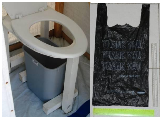
Figure 4: Rapid, low-cost toilet construction (left) by MSF-B for bag (right) used post-EQ in Cité Soliel, Haiti
