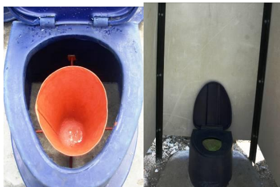
Figure 5: Existing commode with low-cost modification of welded bucket that was the appropriate size of the Peepoo, Port-au-Prince, Haiti
