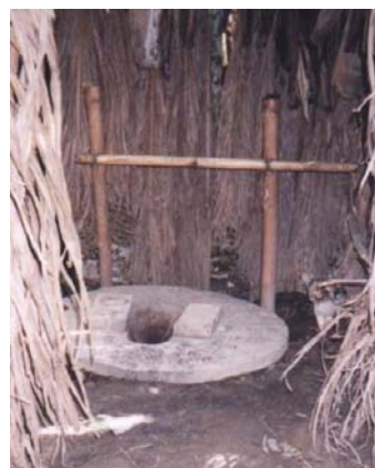
A simple bamboo handrail to help with bending for squatting
