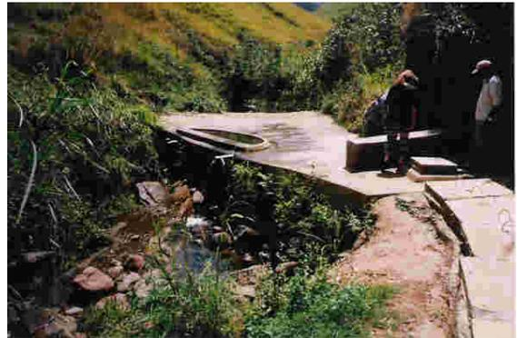
**Spring box with roughing filter on the outlet (to the right) prior to the water entering the pipeline**
