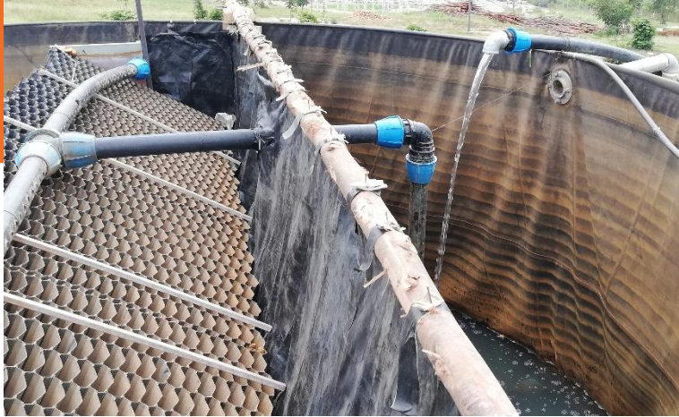
Filling Outlet side of tank with water to ensure structural stability
