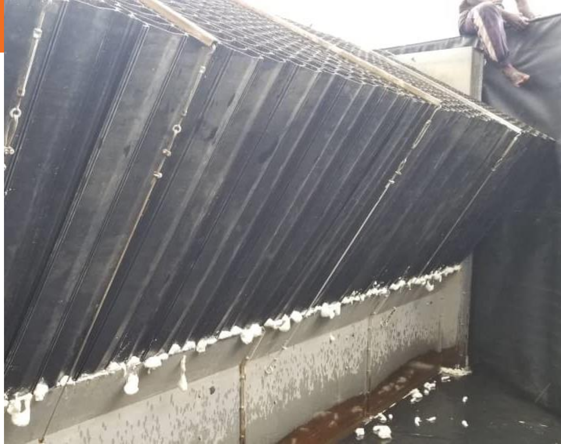
(Above) Bangladesh team solution to reduce leakage along side of tank.
