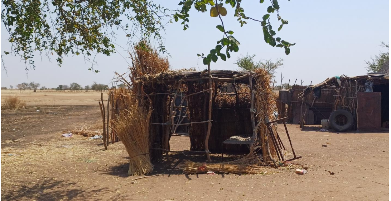
Rakuba shelter under construction, Kueleng Thoi village, Renk, author photo
